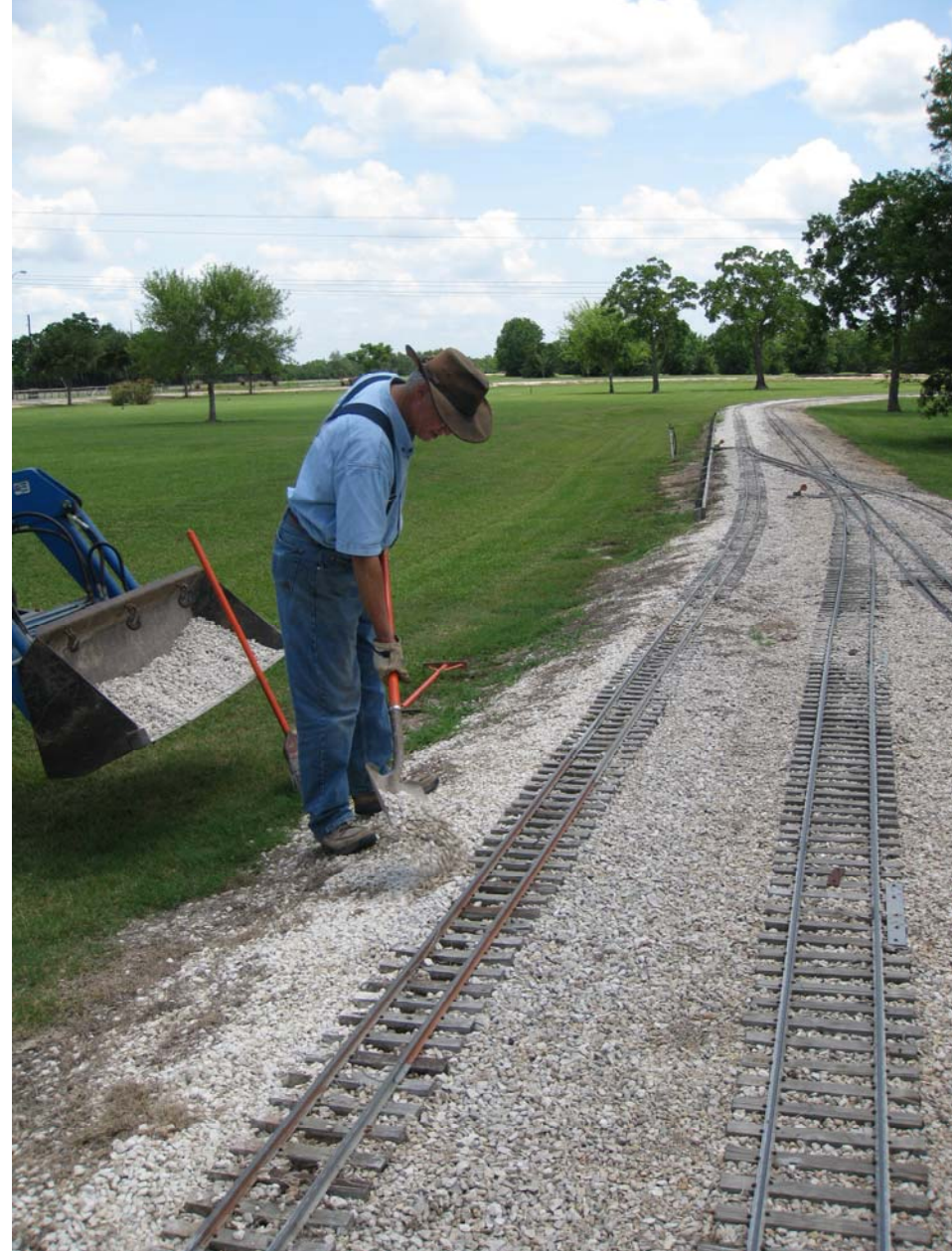
Doug Blodgett tamping (left) and ballasting (right) track.
