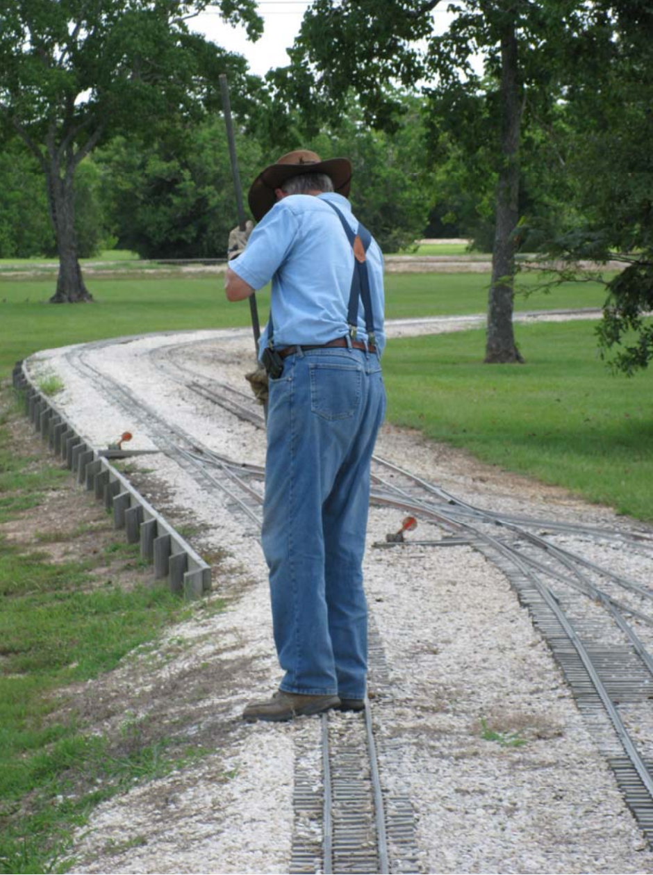
Doug Blodgett tamping (left) and ballasting (right) track.
